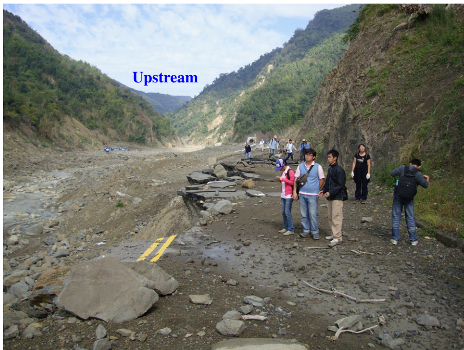
Fig. 5. The slightly damaged road immediately upstream of the landslide dam on the east bank of the Cishan River.
