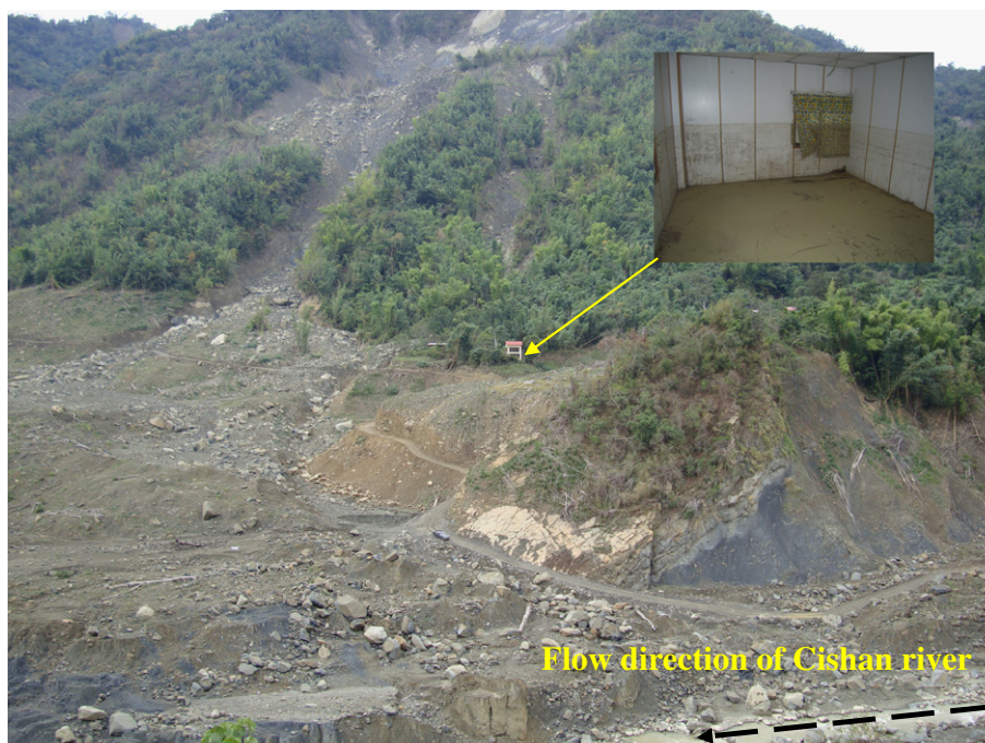
Fig. 7. Water traces were found in a house at about Ele. 440 m. Therefore, the maximum-possible impounded water level of the natural lake was Ele. 440 m.
