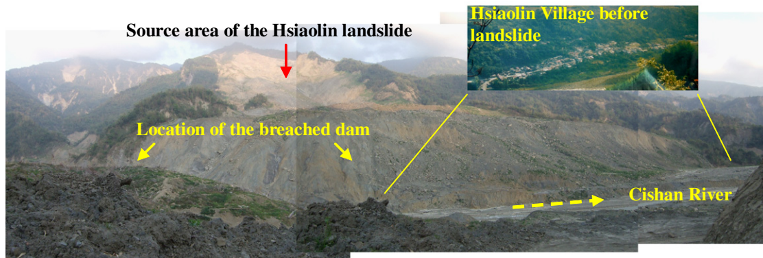
Fig. 1. The Hsiaolin landslide, the landslide dam and the buried Hsiaolin village. The landslide blocked the Cishan River and the landslide dam breached soon after the formation of an impounded lake. Blue line shows the drainage basin upstream of the Hsiaolin SLD. The boundary of the upstream catchment area is generated by the ArchHYDRO tool. The photo was taken from the west bank of the Cishan River shows the breached dam.
