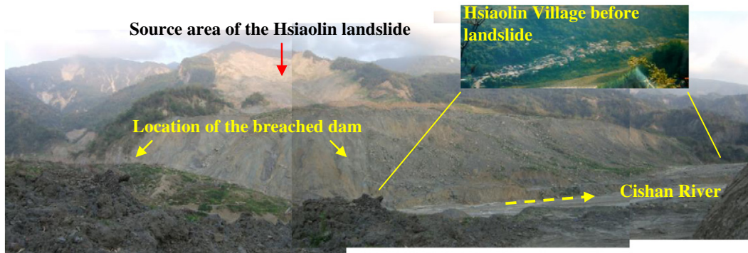
Fig. 1. The Hsiaolin landslide, the landslide dam and the buried Hsiaolin village. The landslide blocked the Cishan River and the landslide dam breached soon after the formation of an impounded lake. Blue line shows the drainage basin upstream of the Hsiaolin short-lived landslide dam. The boundary of the upstream catchment area is generated by the ArchHYDRO tool. The photo taken from the west bank of the Cishan River shows the breached dam.
