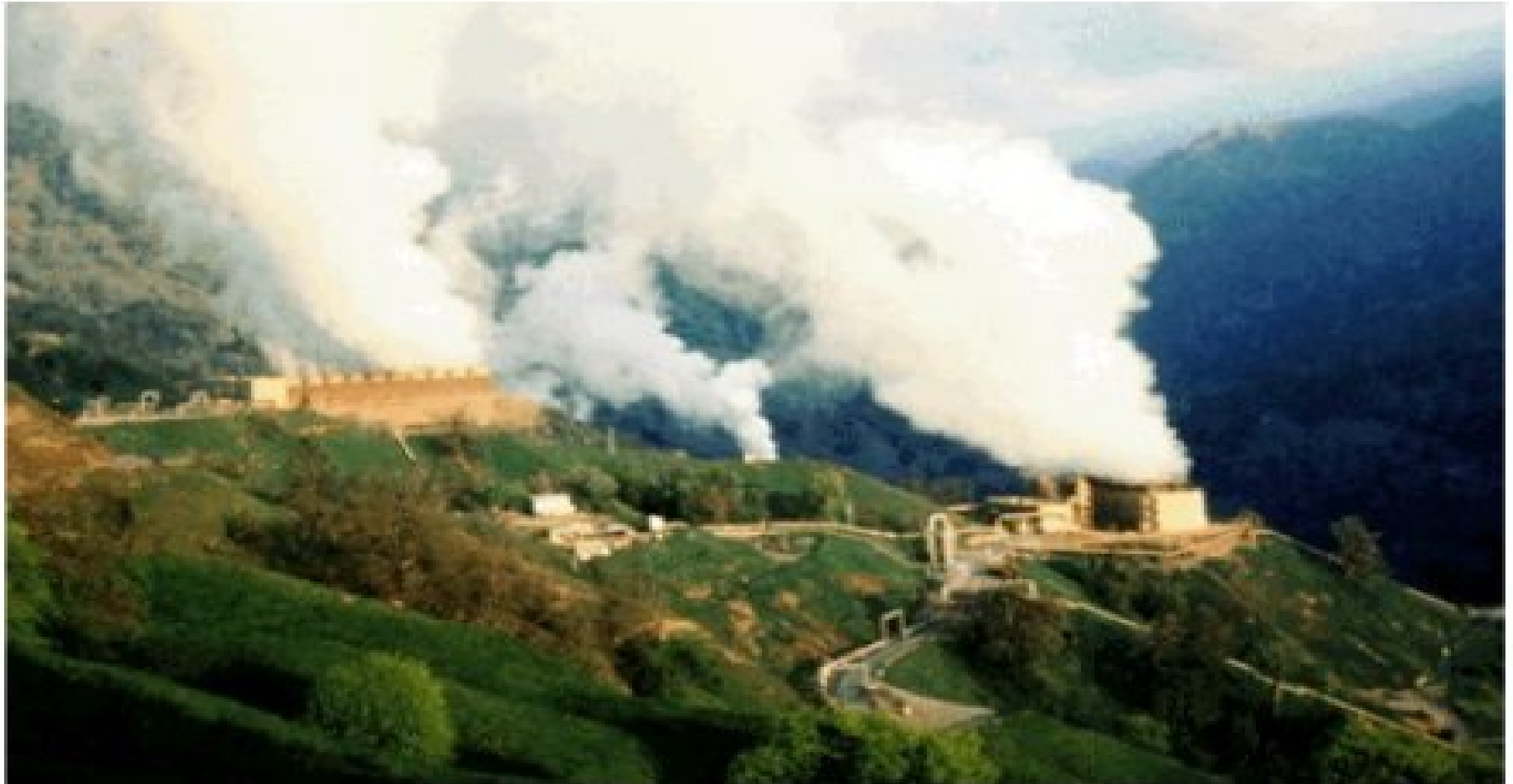
Geothermal plants at the Geysers geothermal field, CA.
