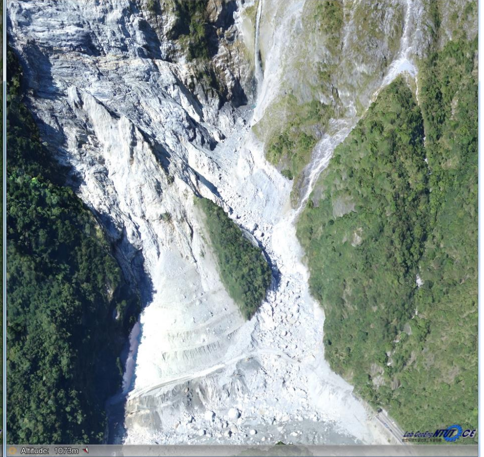
BaiShaBridge after Typhoon
