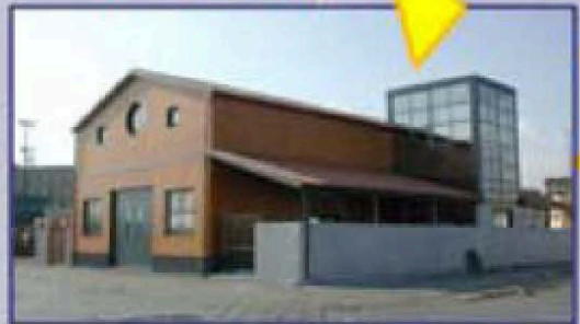
LNS Test Site Laboratory at the port of Catania
