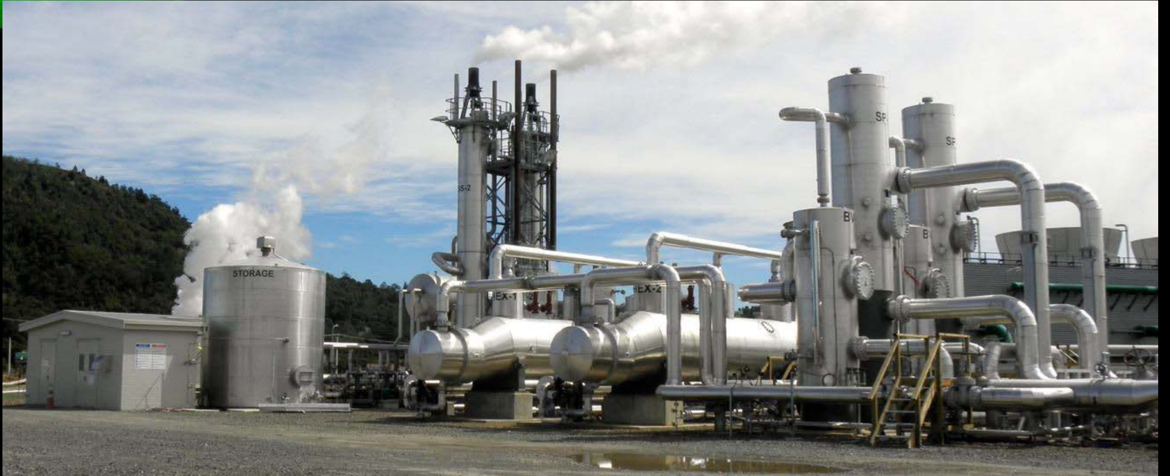
Clean steam plant, Kawerau geothermal plant, Taupo, New Zealand
