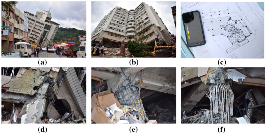
Fig. 8 a Front view, b back view, c drawing of floor plan, d corner column, and e and f bottom columns of the collapsed 12-story mixed-use apartment block
