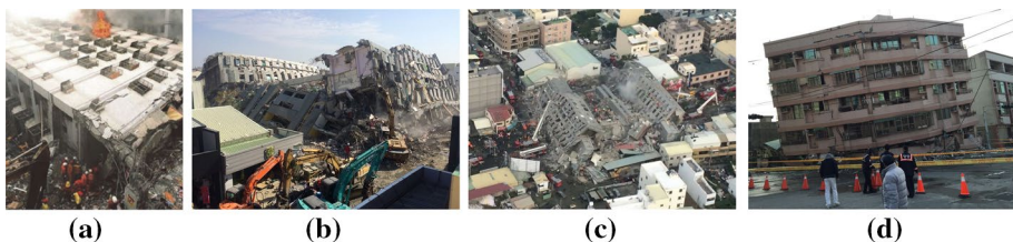
Fig. 20 a A 12-story building collapsed during the 1999 Chi-Chi earthquake, b a 16-story building collapsed during the 2016 Meinong earthquake, c a bird's eye view of the collapsed building shown in b , d a 7-story building collapsed during the 2016 Meinong earthquake
